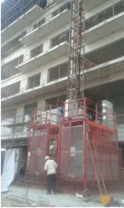
Construction hoist in operation
