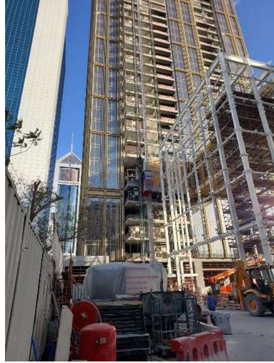
Hoist installation on a high-rise tower
