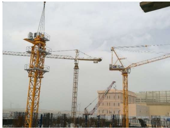
Multiple tower cranes on site
