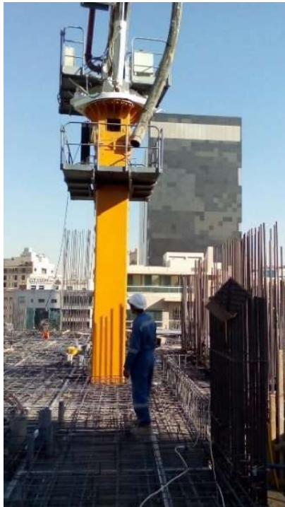
Concrete placing boom in operation
