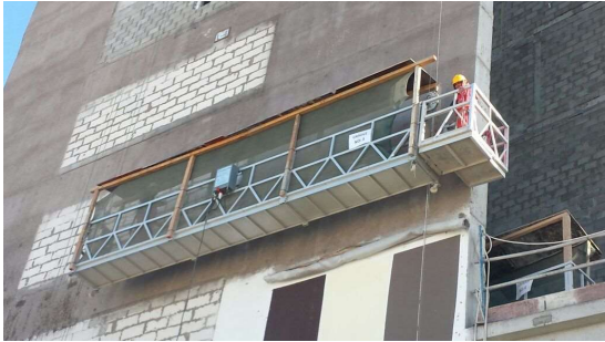
Cradle deployed on a building façade
