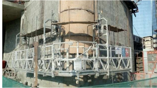
Cradle deployed on an industrial structure
